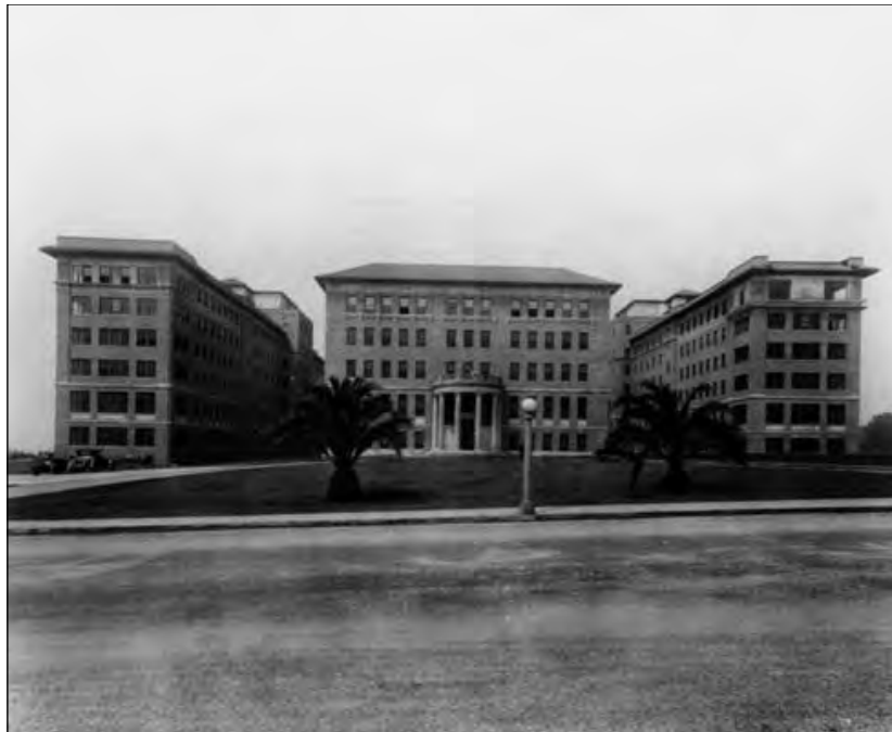
Figure 98: Subarea 7—General Hospital, Wadsworth Hospital (not extant) under construction, view west (Los Angeles Public Library, circa 1925)
