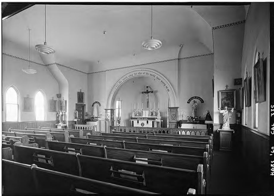
Figure 42: Subarea 1: Domiciliary, Chapel, Catholic Chapel (HABS CAL,19-LOSAN,12A-1, 1960)
