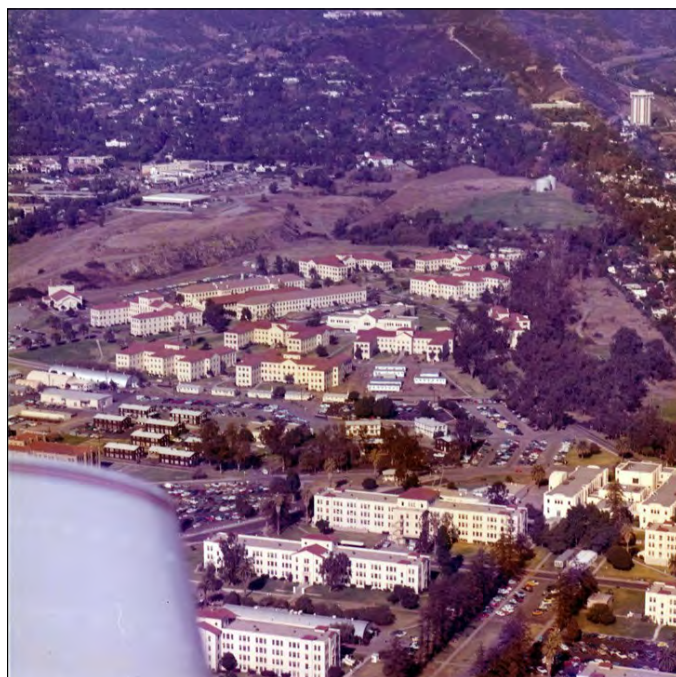
Figure 58: Subarea 1: Domiciliary (bottom right ) and subarea 4—Neuropsychiatric (N.P.) Hospital (top left), view northwest (VA Archives, circa 1984)
