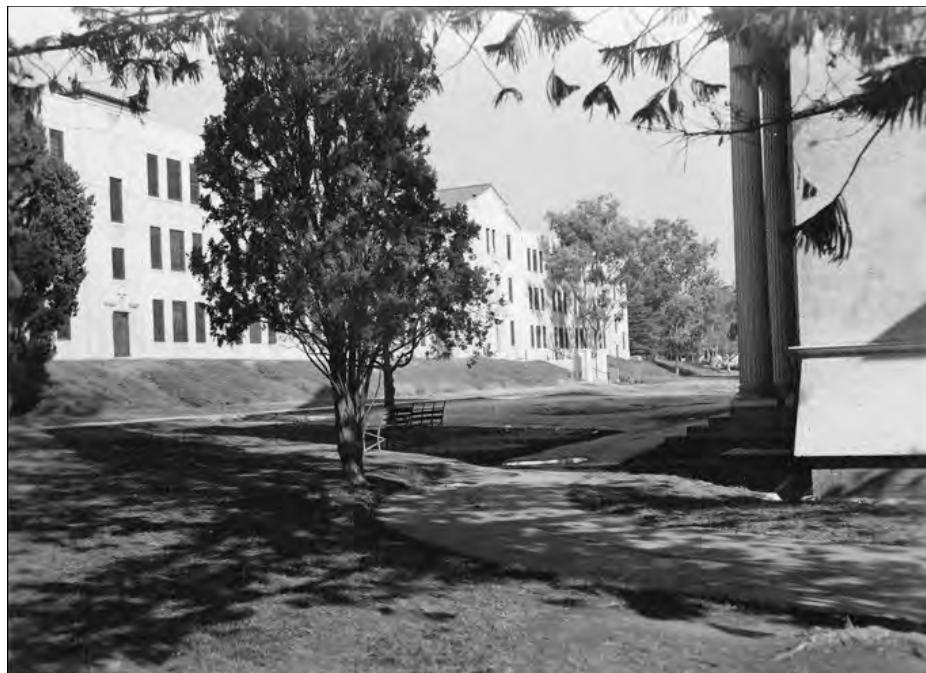
Figure 44: Subarea 1—Domiciliary, Second generation domiciliary building (extant), view northeast (VA Archives, nd)
