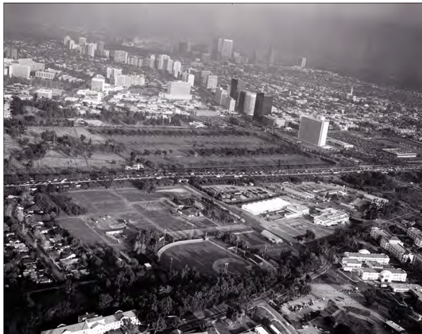
Figure 93: Subarea 5—Utility, view southeast (VA Archives, circa 1984)
