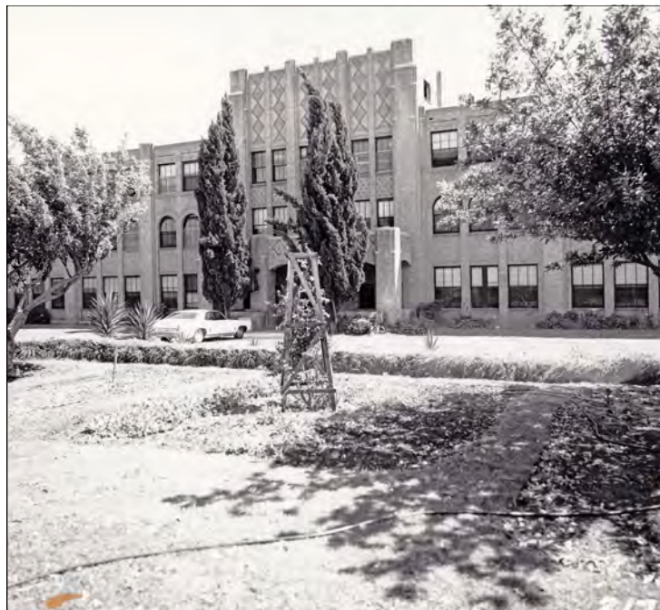
Figure 65: Subarea 3—Research, Building 116, view northwest (VA Archives, nd)
