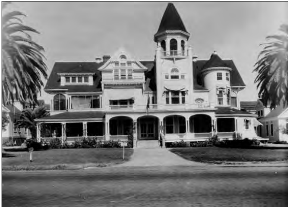
Figure 27: Subarea 1—Domiciliary, Barrack #6 (not extant), view east (Los Angeles Public Library, circa 1923)
