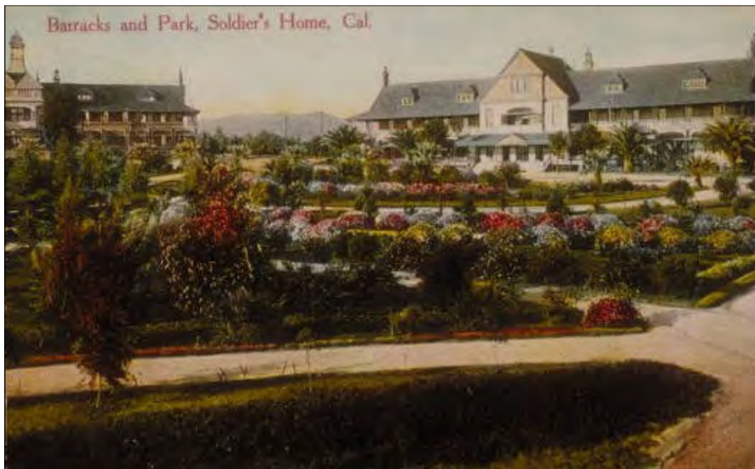
Figure 7: Subarea 1—Domiciliary, Barracks #4 (left, not extant) and #5 (right, not extant), view northeast (Santa Monica Public Library, 1890)
