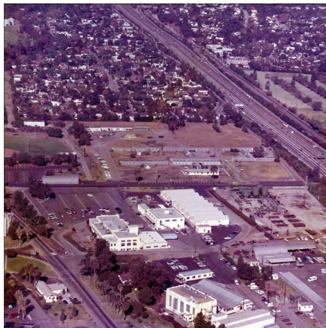
Figure 94: Subarea 5—Utility, view north (VA Archives, circa 1984)
