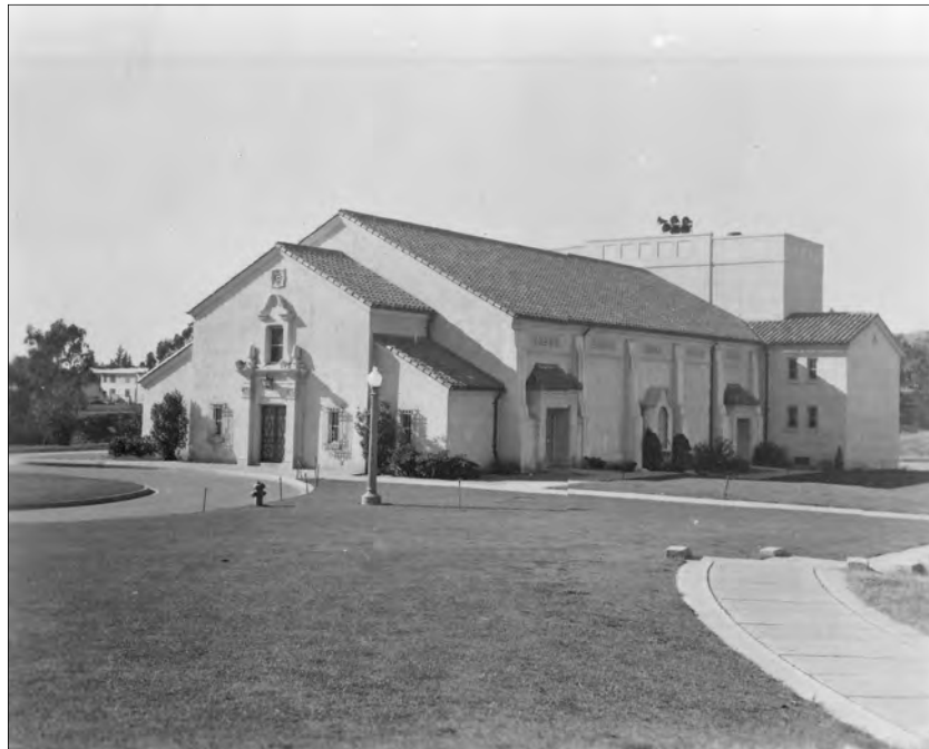
Figure 73: Subarea 4—Neuropsychiatric (N.P.) Hospital, Building 211, Brentwood Theater (extant), view southwest (VA Archives, nd)
