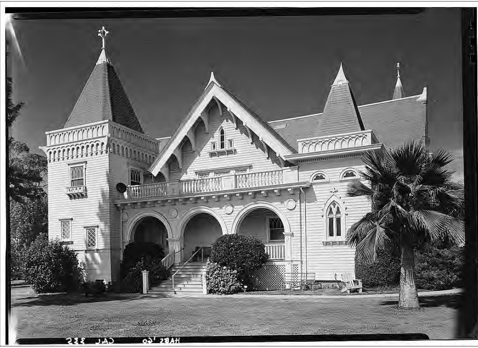
Figure 40: Subarea 1—Domiciliary, Chapel, view north (HABS CAL,19-LOSAN,12A-1, 1960)
