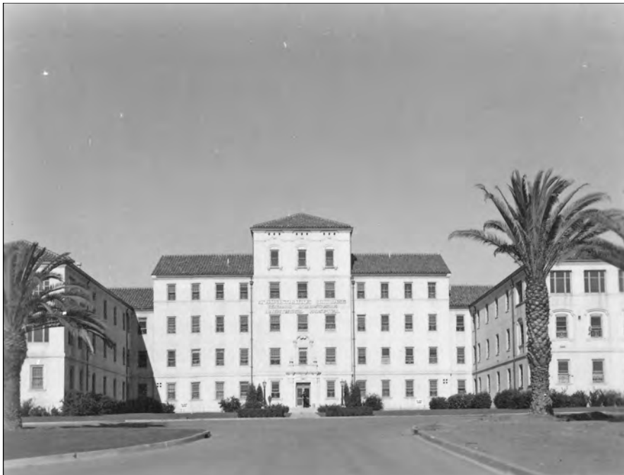
Figure 76: Subarea 4—Neuropsychiatric (N.P.) Hospital, Building 258 (extant), view north (VA Archives, nd)
