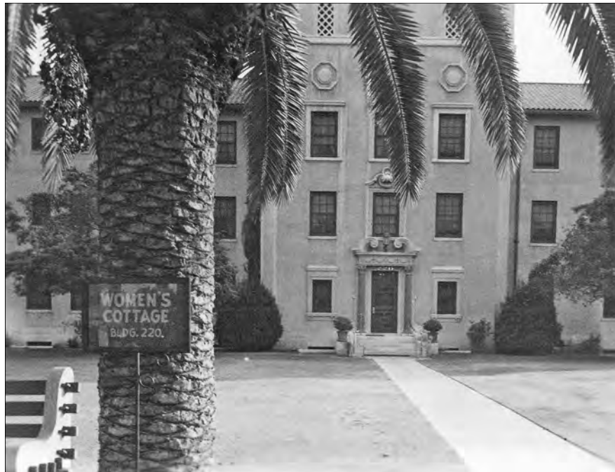
Figure 47: Subarea 1—Domiciliary, Building 220, Women's Cottage (extant), view south (VA Archives, nd)
