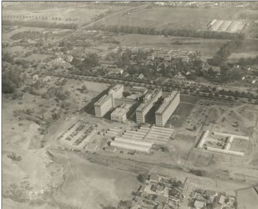
Figure 102: Subarea 7—General Hospital, Wadsworth Hospital (not extant), view northeast (VA Archives, circa 1965)
