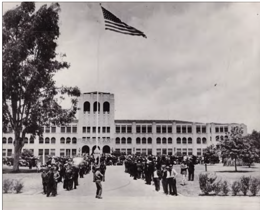
Figure 63: Subarea 3—Research, Building 114, view northeast (VA Archives, nd)
