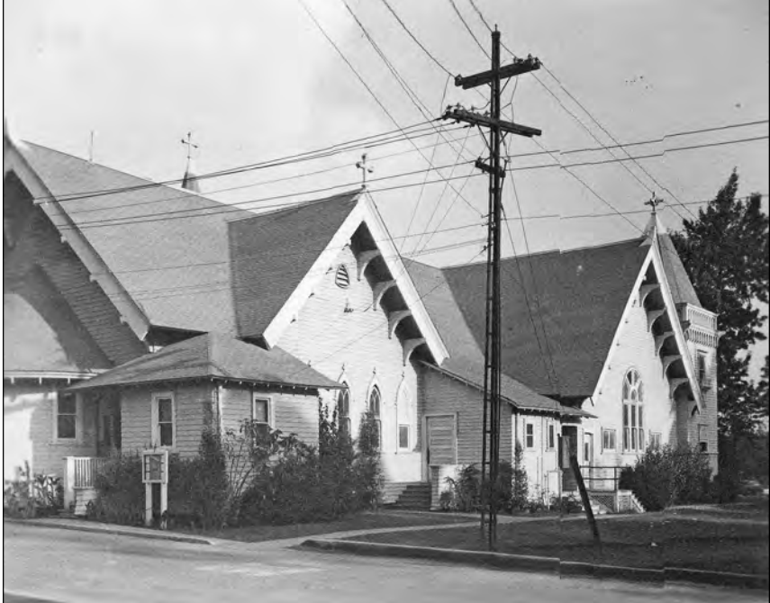
Figure 37: Subarea 1—Domiciliary, Chapel, view northwest (VA archives, nd)
