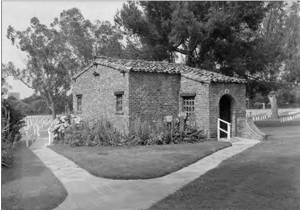
Figure 123: Cemetery, Comfort Station (restrooms, HABS No. CA 2709-26, 2000)
