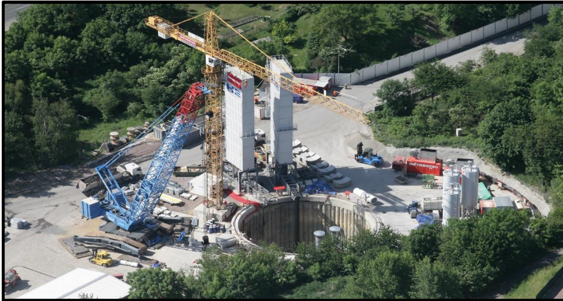
Figure 2-3: Tower Crane and Vertical Conveyor Belt Storage Towers (Example)
