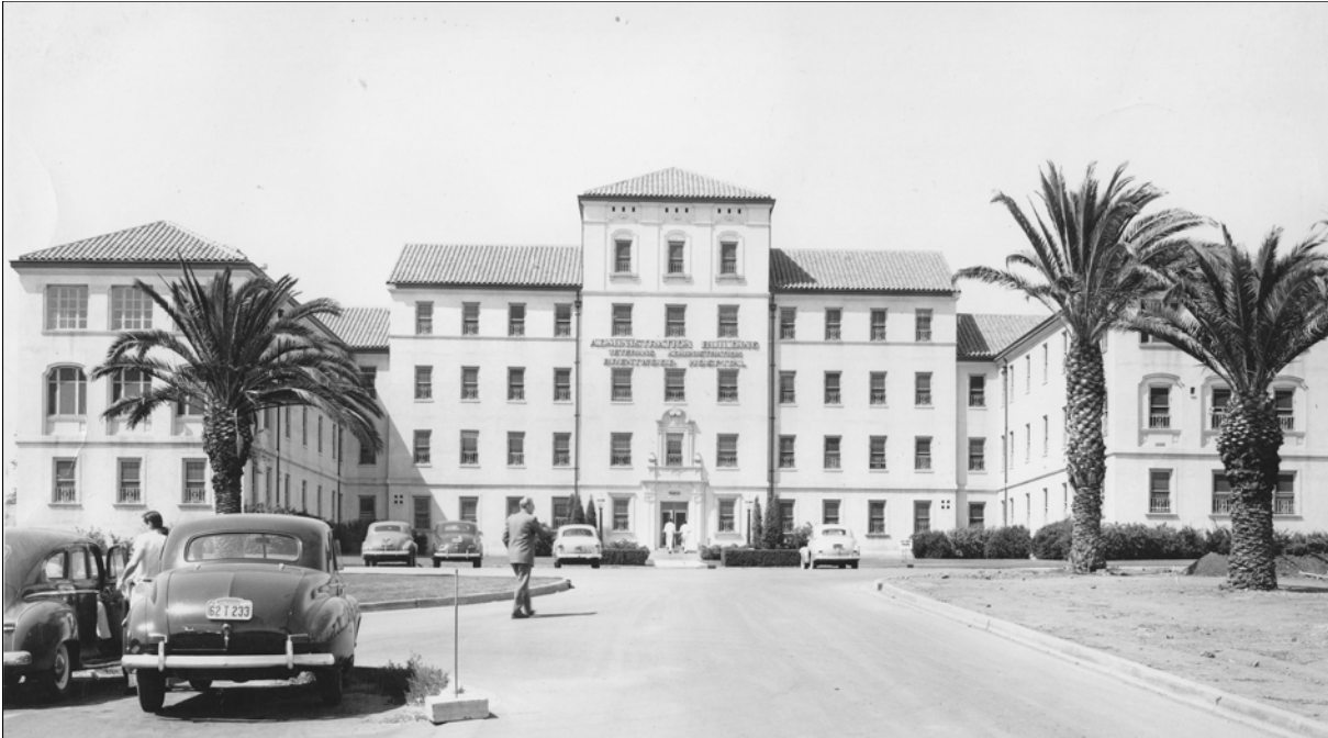
Figure 75: Subarea 4—Neuropsychiatric (N.P.) Hospital, Building 258 (extant), view northwest (VA Archives, circa 1950s)
