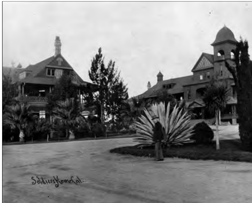
Figure 17: Subarea 1: Domiciliary, Barrack #3 (left, not extant) and #1 (right, not extant), view northwest (Los Angeles Public Library, 1895)
