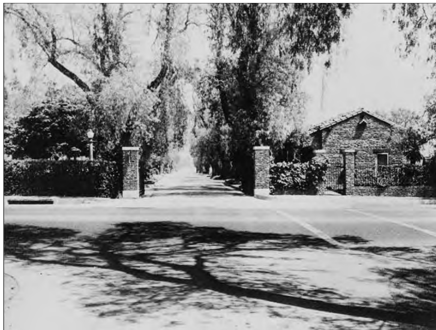
Figure 109: Cemetery, entrance gate with gatehouse (not extant, HABS No CA-2709-B-2, 1949)
