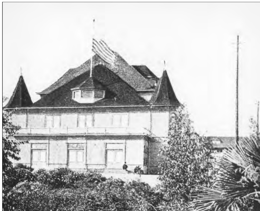
Figure 34: Subarea 1—Domiciliary, Memorial Hall (not extant), view south (VA Archive, nd)
