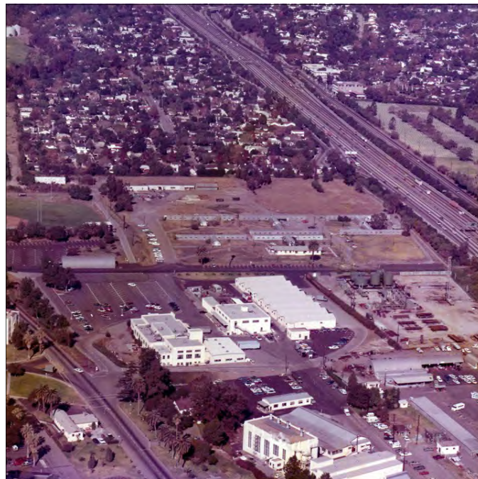
Figure 94: Subarea 5—Utility, view north (VA Archives, circa 1984)
