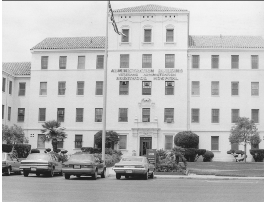
Figure 77: Subarea 4—Neuropsychiatric (N.P.) Hospital, Building 258 (extant), view northwest (VA Archives, circa 1980s)
