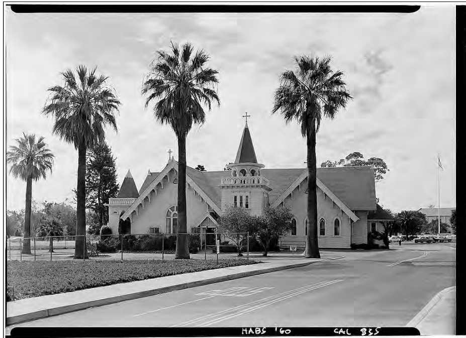
Figure 39: Subarea 1—Domiciliary, Chapel, view west (HABS CAL,19-LOSAN,12A-1, 1960)
