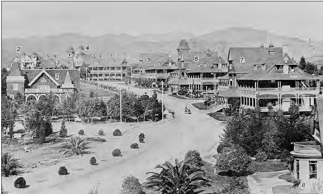
Figure 5: Subarea 1—Domiciliary, view northwest along Bonsall Avenue (HABS CAL,19-LOSAN,12B-1, 1902, reprinted 1963)
