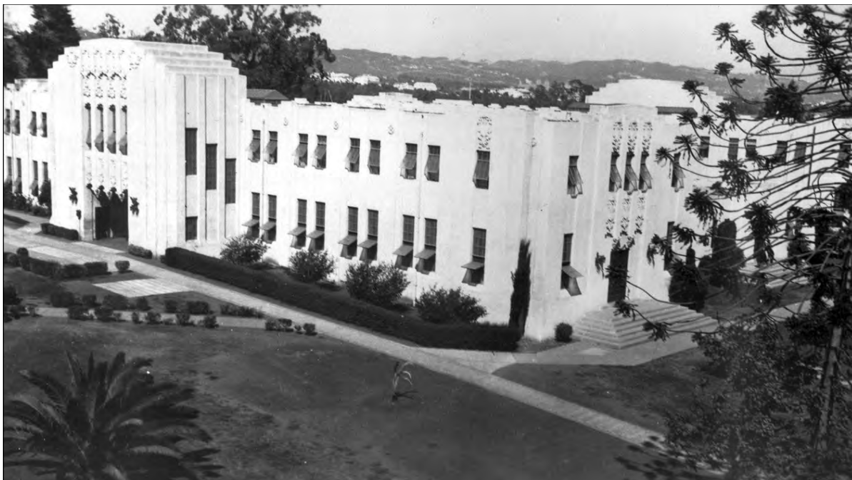
Figure 46: Subarea 1—Domiciliary, Building 13, General Mess Hall (extant), view northwest (VA Archives, nd)
