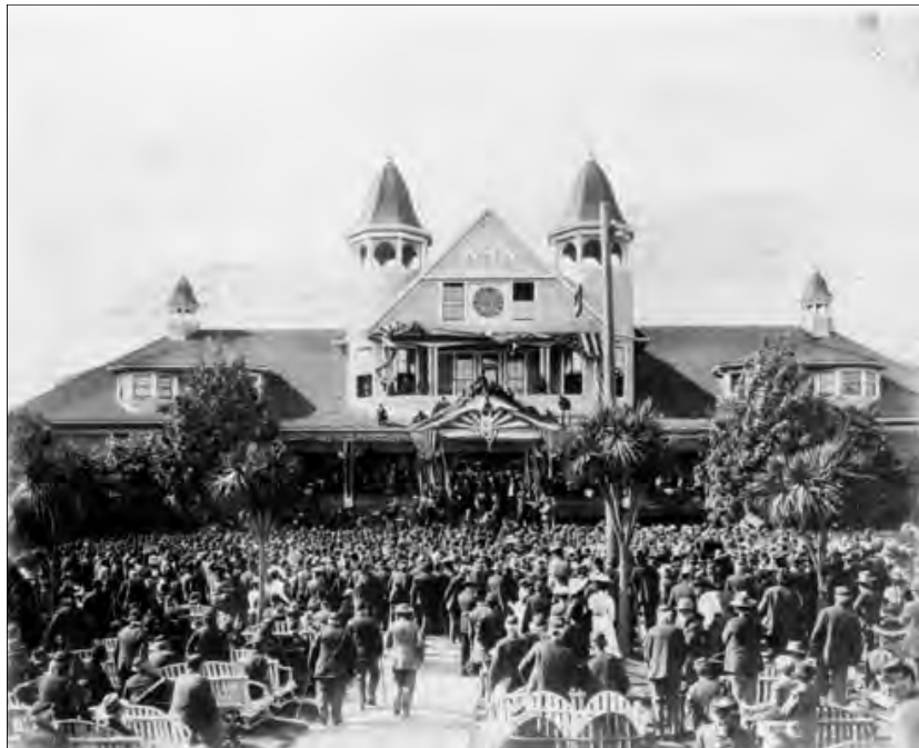
Figure 12: Subarea 1—Domiciliary, Assembly Hall (not extant), visit from President McKinley, view north (Los Angeles Public Library, 1901)
