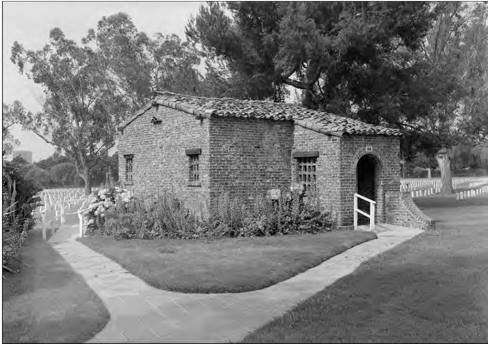
Figure 123: Cemetery, Comfort Station (restrooms, HABS No. CA 2709-26, 2000)
