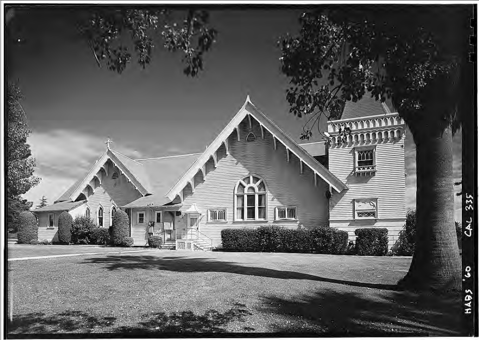
Figure 38: Subarea 1—Domiciliary, Chapel, view west (HABS CAL,19-LOSAN,12A-1, 1960)
