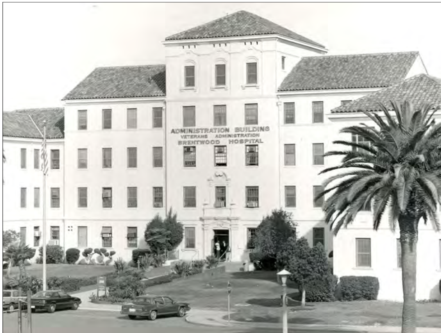
Figure 78: Subarea 4—Neuropsychiatric (N.P.) Hospital, Building 258 (extant), view northwest (VA Archives, circa 1980s)
