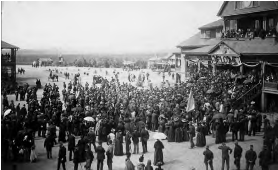
Figure 15: Subarea 1—Domiciliary, Assembly Hall (right, not extant), view west (Los Angeles Public Library, 1892)
