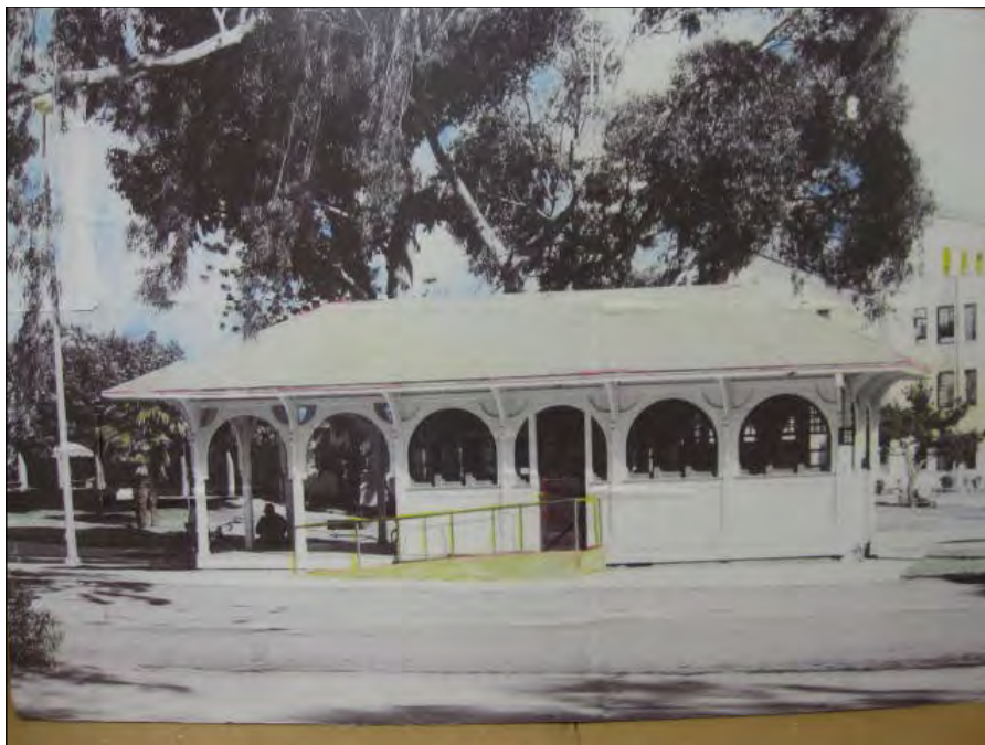
Figure 48: Subarea 1—Domiciliary, Building 66, Trolley House (extant), view north (VA Archives, nd)
