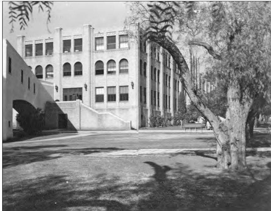
Figure 66: Subarea 3—Research, Building 113, view northeast (VA Archives, nd)
