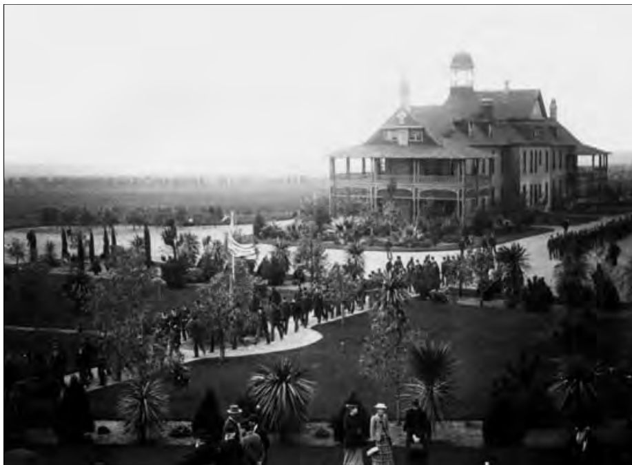
Figure 16: Subarea 1—Domiciliary, Barrack #3, view west (Los Angeles Public Library, 1892)
